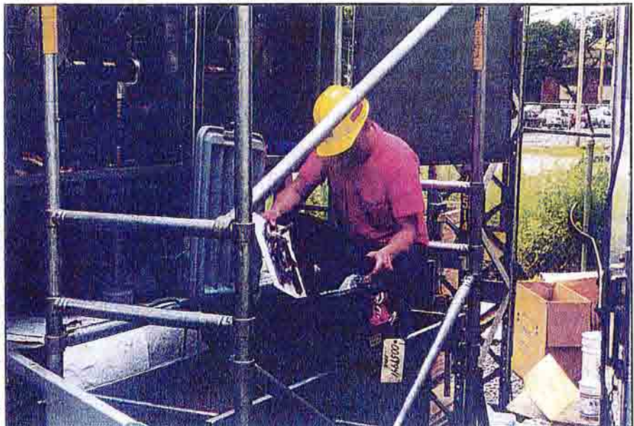
Fig. 2. An RG&E technician using the kit to repair an LTC.
